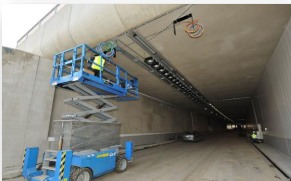
Leopold III-tunnel Brussel
